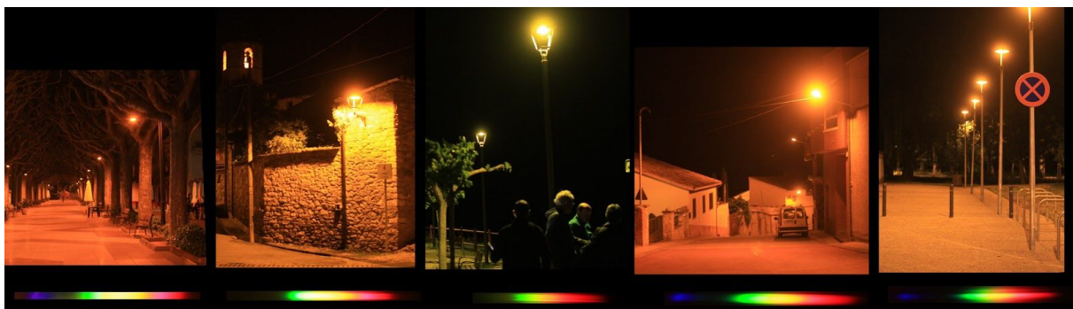
Figure 51: Tremp, Rambla Dr. Pearson (PC amber), Guardia de Noguera (amber filtered LED), Guardia de Noguera (green-yellow filtered LED), Les Avellanes (PC amber), Banyoles (PC amber Ignialight).
